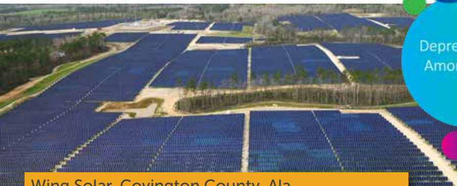
Wing Solar, Covington County, Ala.
